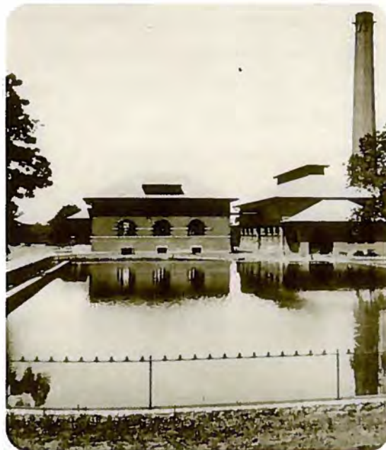
Coal burning power plant. 1896
